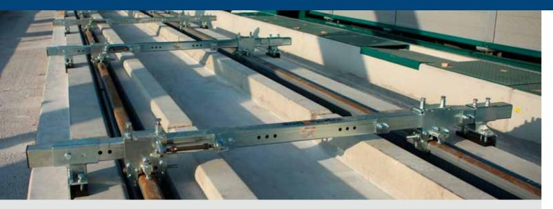
Installation and geometric alignment of the rails take place in accordance with the two techniques described below (Top-Down and Bottom-Up). For the embedding work, either project-dedicated machines pour the Corkelast®, or it is applied by manual pouring from buckets.
